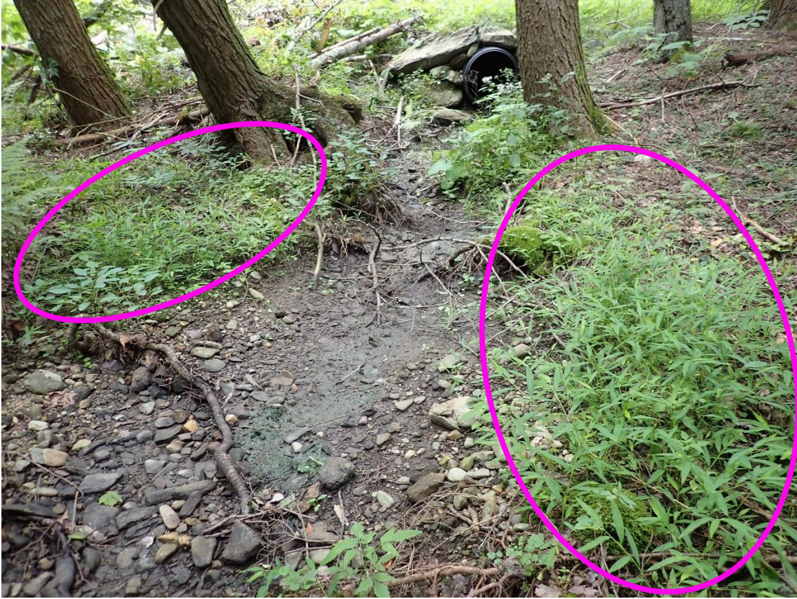
Photo 3: This photo of the existing conditions at 648 East St. supports the connection between the culvert, stormwater runoff and Japanese stilt grass infestations. This connection can be clearly observed by the stilt grass populations in the above photo circled in pink.
