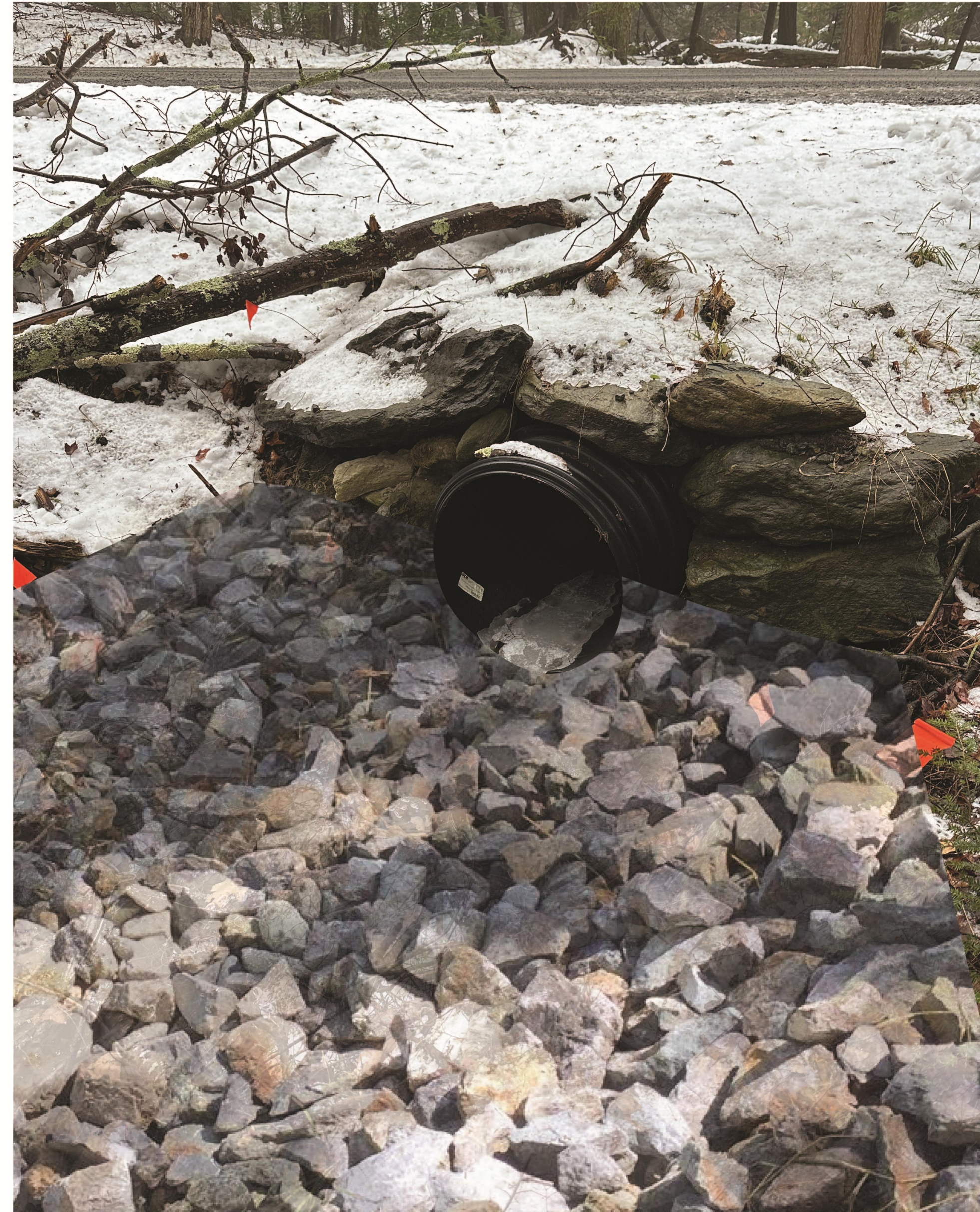
PROPOSED CONDITION: STONE OUTLET PROTECTION
